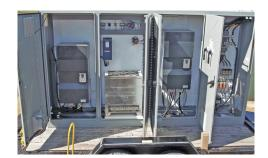
MOTOR STARTER PANEL. The motor starter panel provides options to configure a control system that best fits your application – whether that's a soft-start or VFD panel.
